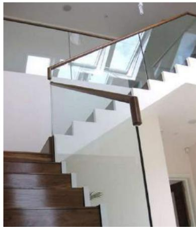
DJ Panel to be designed to project approx 300mm over stairwell and be secured to balustrade. This will help with access. Modern glass panels (no curves).
